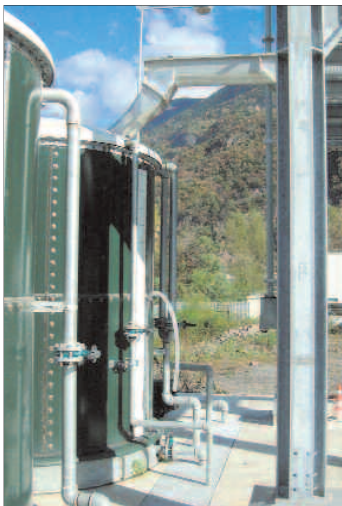
Detail of the dissolution system with automatic salt metering screw
