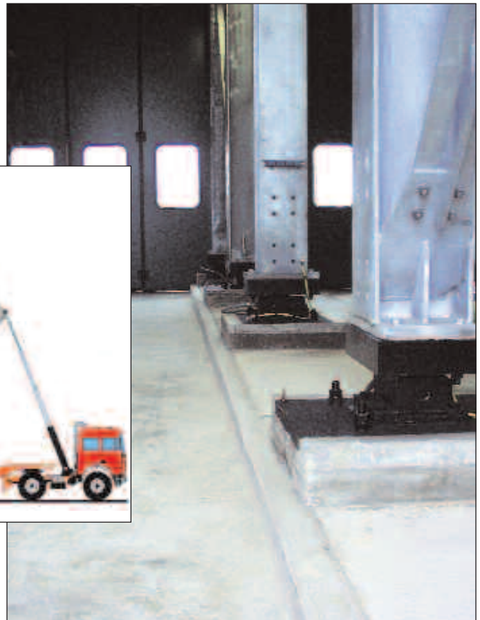
The load cell and positioning under the columns
