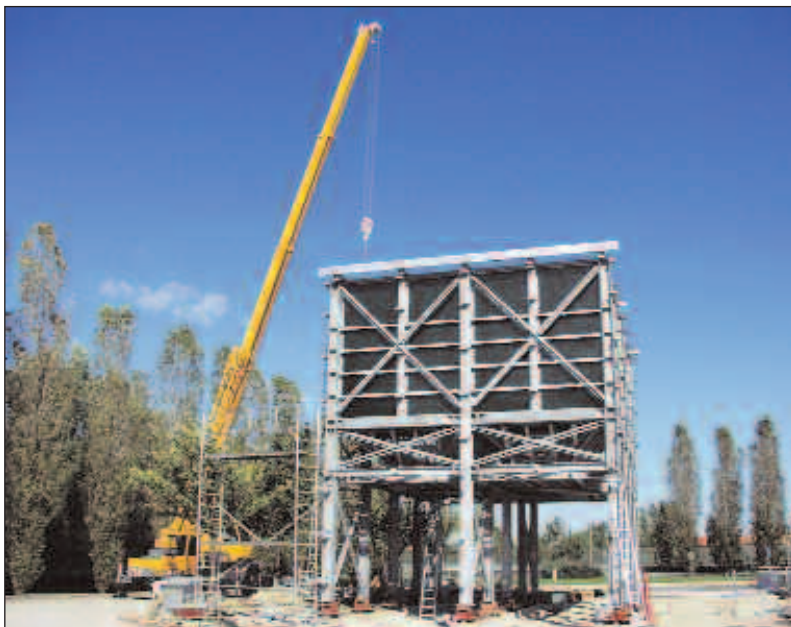
The load bearing structure of the silos in the installation phase
