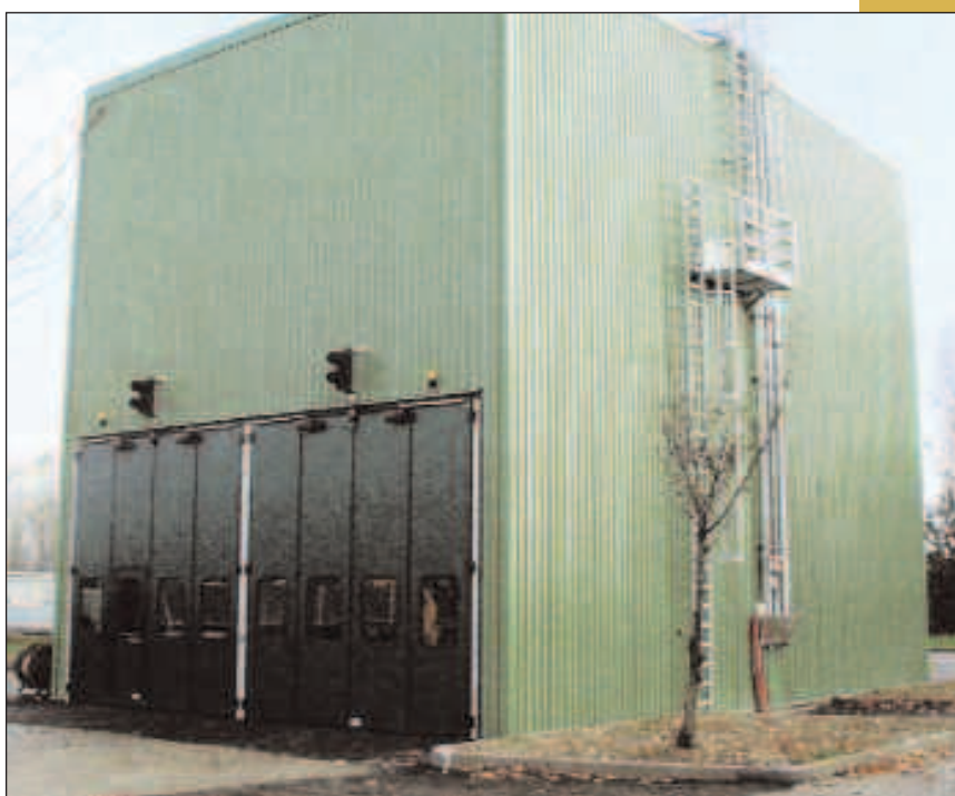
The 500-tonne modular salt storage facility with low environmental impact
