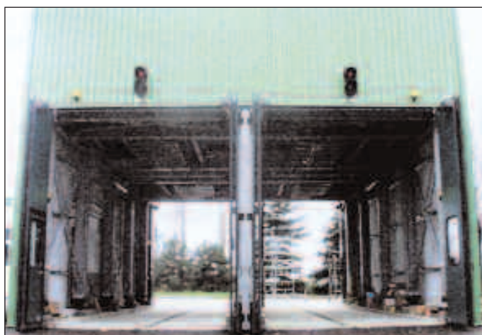
A view of the passageways for loading vehicles
